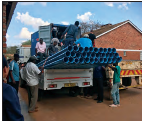
Lions build water wells for communities in Malawi, enabling residents to get safe drinking water
