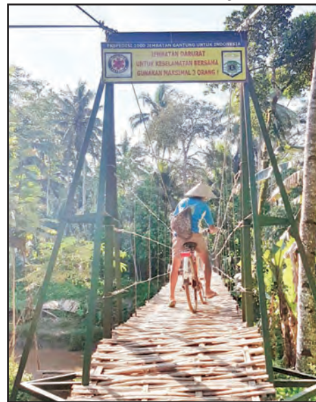
A villager crosses the newly constructed hanging bridge
