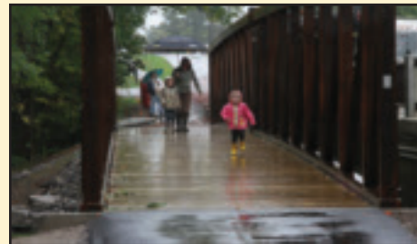
Complete and usable. Installed on Saturday September 21, 2013 during 5 hours of rain
