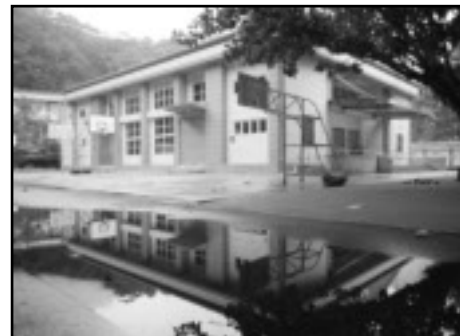
The shelter at the junior high is strong enough to withstand an earthquake
