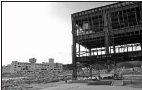
Office buildings in Minami Sanriku are ruined
