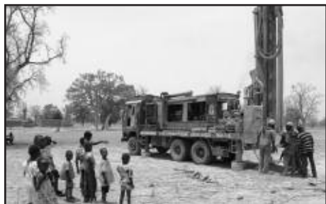
A crew digs the new well for Dissan, Mali
