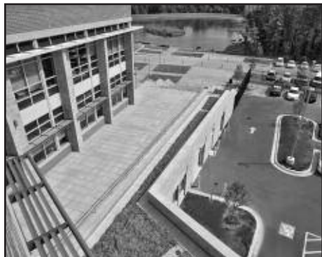
The Bowie city hall has a green roof and recycled materials in its brick, steel and concrete
