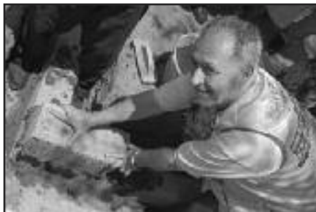
International Director Roberto Fresia of Italy lays the cornerstone for a health facility in Zambia
