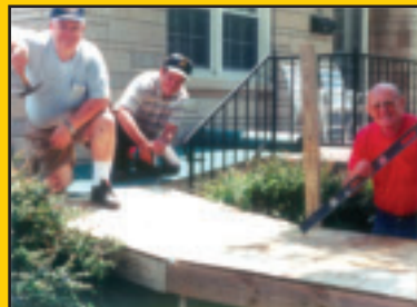
Lions from Bedford, Indiana build a wheelchair ramp.
